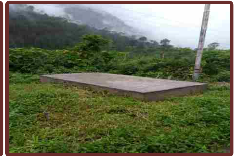
Foundation for DG set
