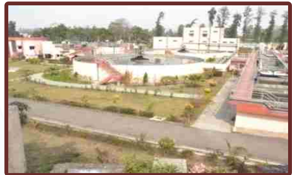
27 MLD STP AT JAGJEETPUR, HARIDWAR
