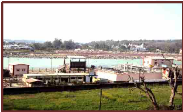
3 MLD STP AT SWARGASHRAM
