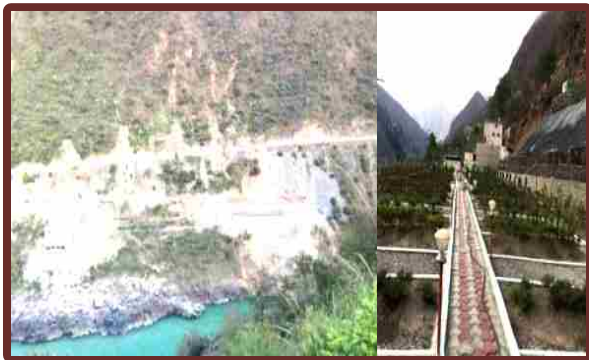
1.4 MLD STP AT DEVPRAYAG
