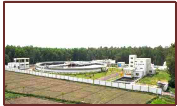
18 MLD STP AT SARAI, HARIDWAR
