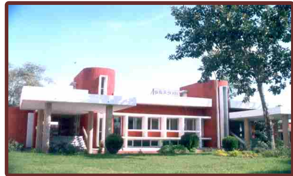
MAIN SEWAGE PUMPING STATION, JAGJEETPUR
